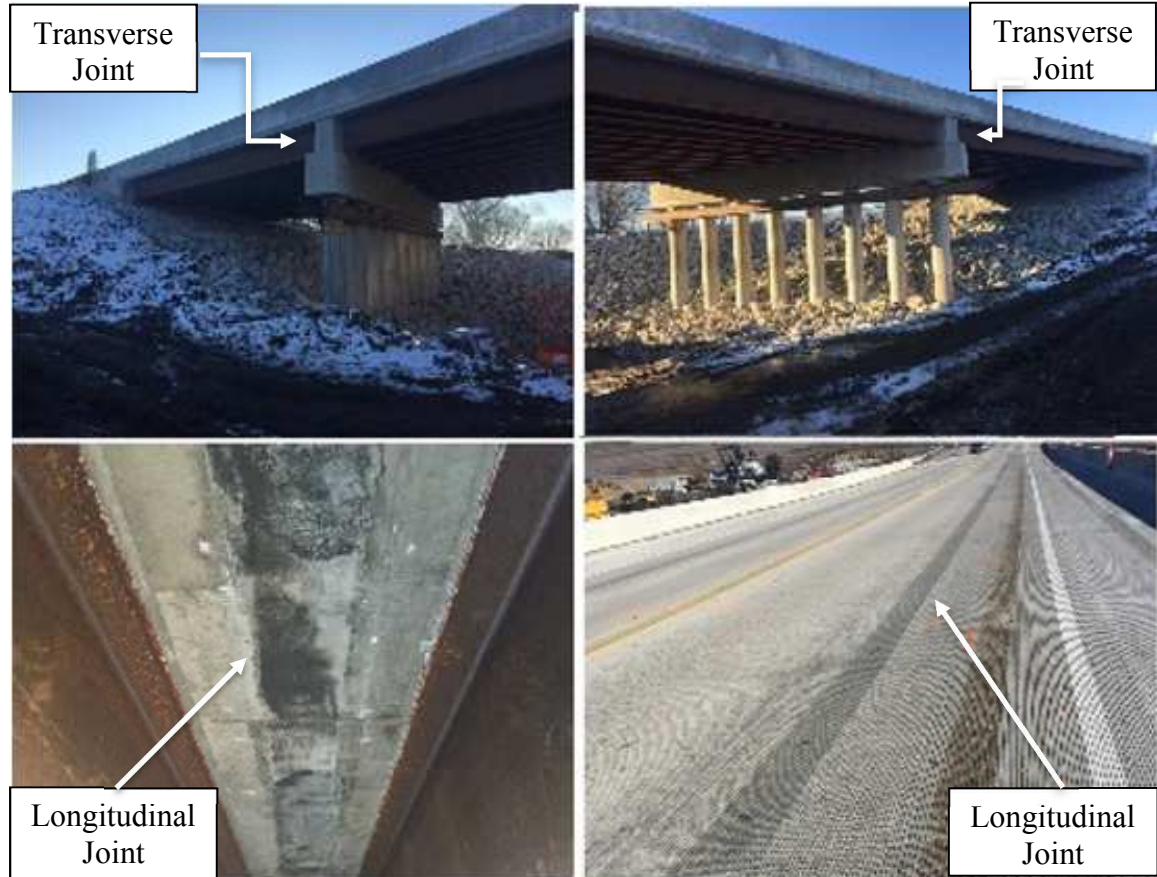
Figure 3-3. Constructed Little Silver Creek Bridge
