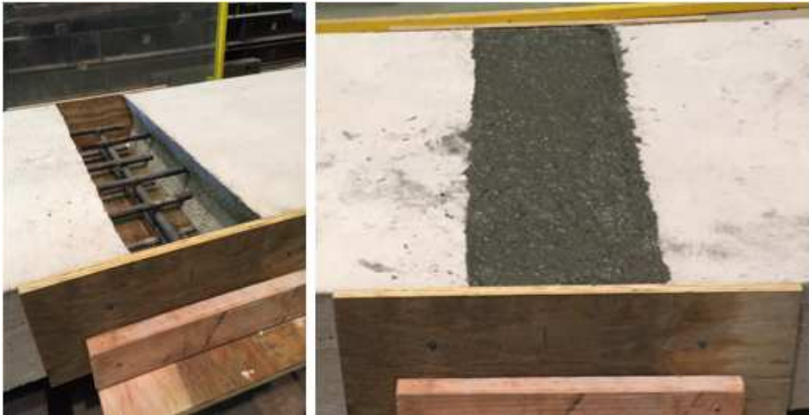
Figure 3-14. Formwork Construction and Placement of Joint Material
