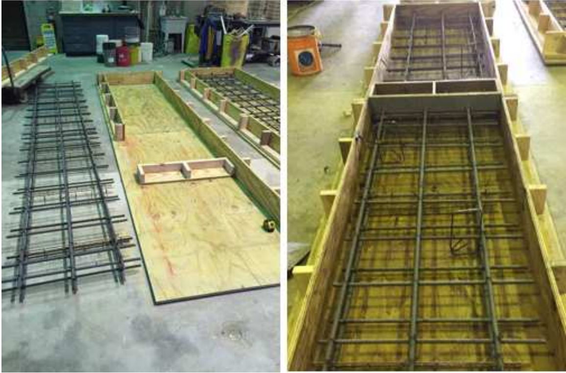
Figure 3-11. Steel Reinforcement and Formwork Fabrication
