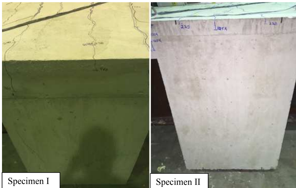
Figure 4-20. Diaphragm Cracks on Long Side for Each Specimen
